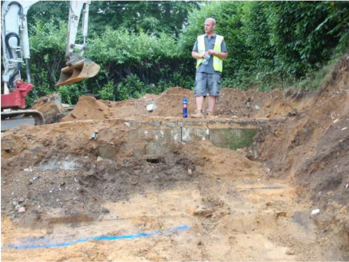
Plate 4. Ground reduction and removal of existing building (facing south-west)
