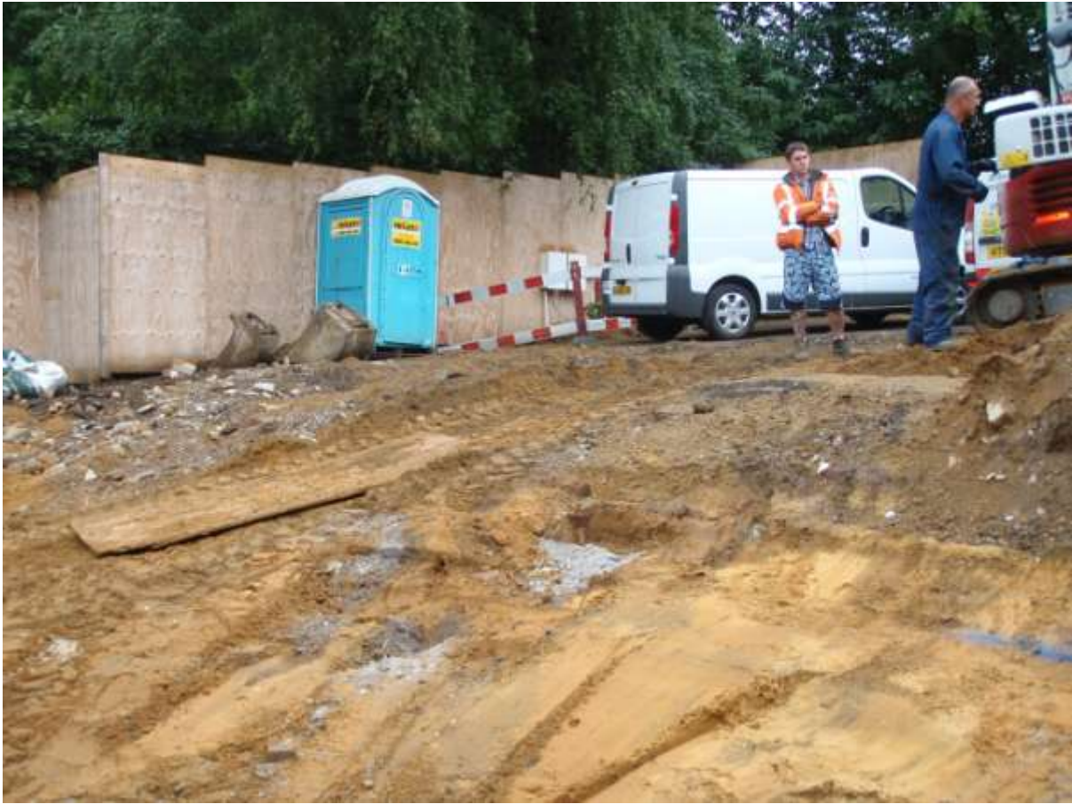
Plate 3. The site (facing west)
